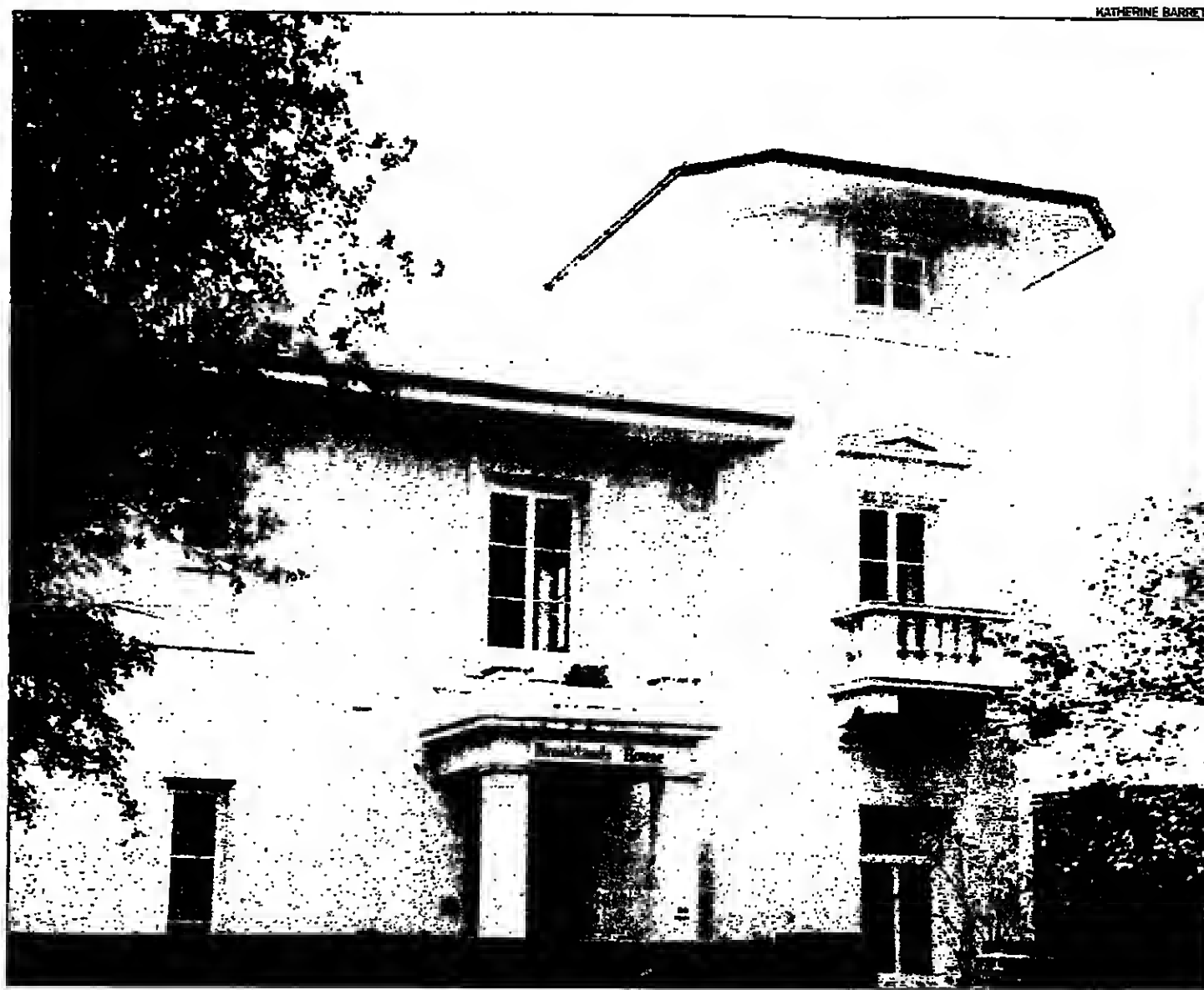
BROOKLANDS HOUSE was built by George Smith in 1826 when he was surveyor to the Cator family, the local landlords after whom the estate is named. Now its turret apartment is for sale at £199,950. Brooklands, used as a family house until 1918, passed into social club use and tennis courts were built in its large
